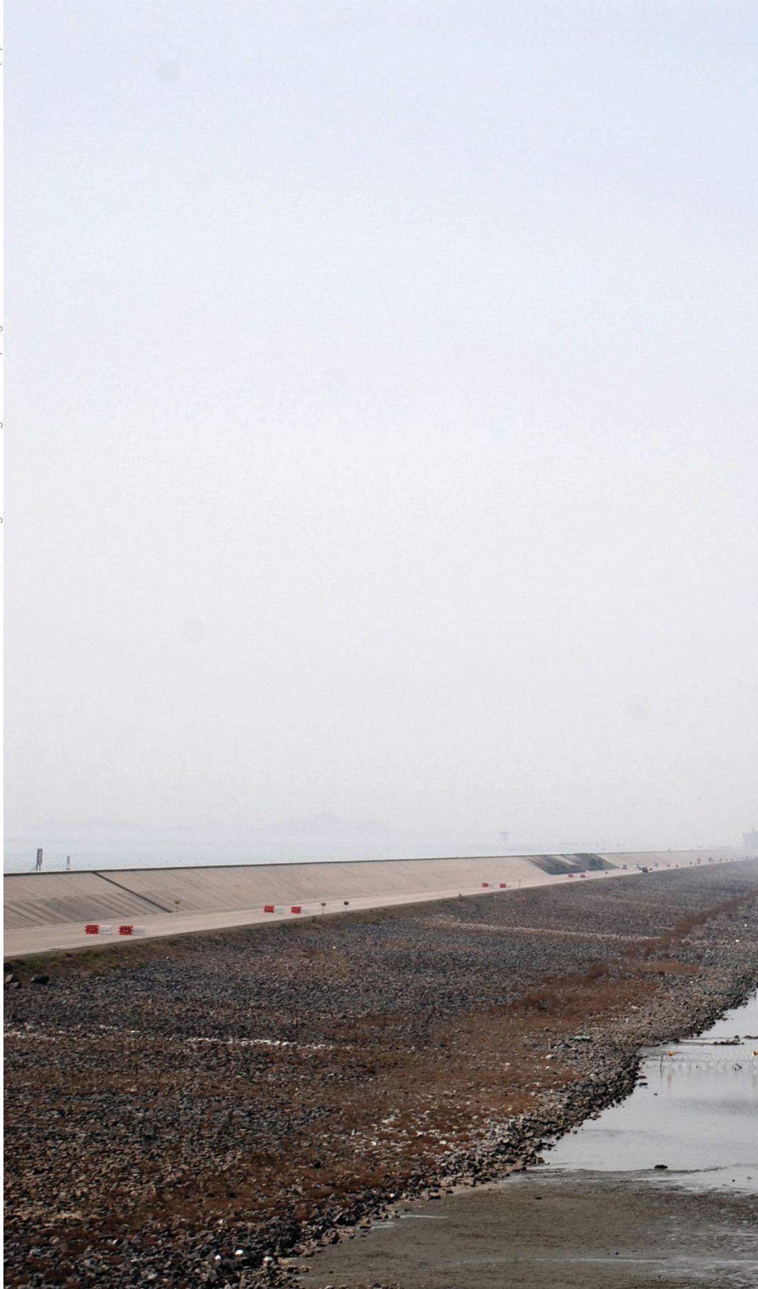
View looking towards the Gogunsan Archipelago from the south end of the sea wall. Alex Bank, April 2008
